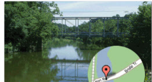
Station Road Bridge
